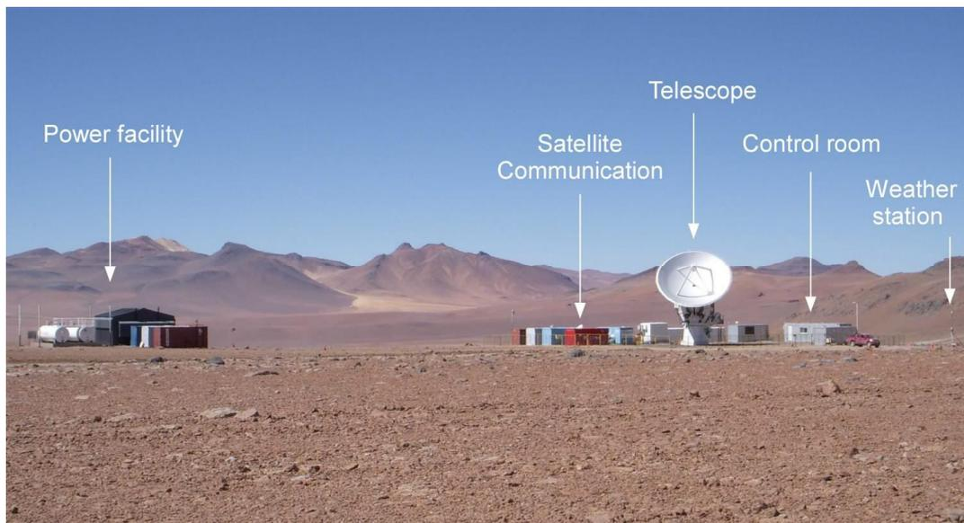
Fig. 3 The current view of the ASTE infrastructure at Pampa la Bola. Several key facilities are surrounding the telescope, including the electrical power facility, containers for telescope control, small lab to prepare the receivers, weather station, and a satellite communication system.
